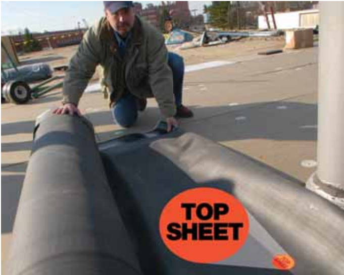
Locate the orange "TOP SHEET" Sticker on 2-packs to ensure proper roll-out.
